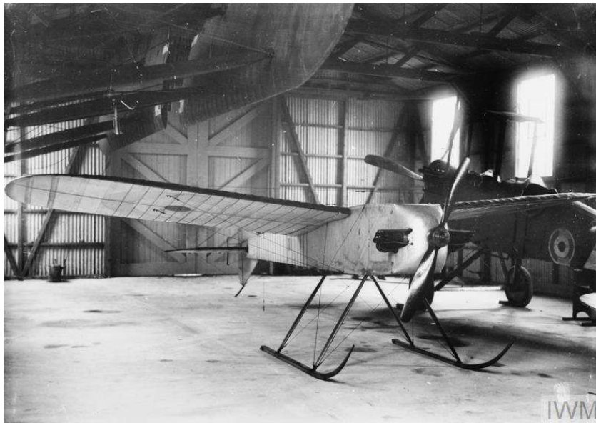
Figure 2: Aerial Target from the First World War (IWM's collection)
